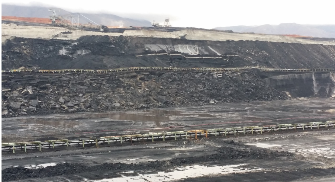
Figure 9. Local slope failure due to detachment of lignite from marl in the fault zone
