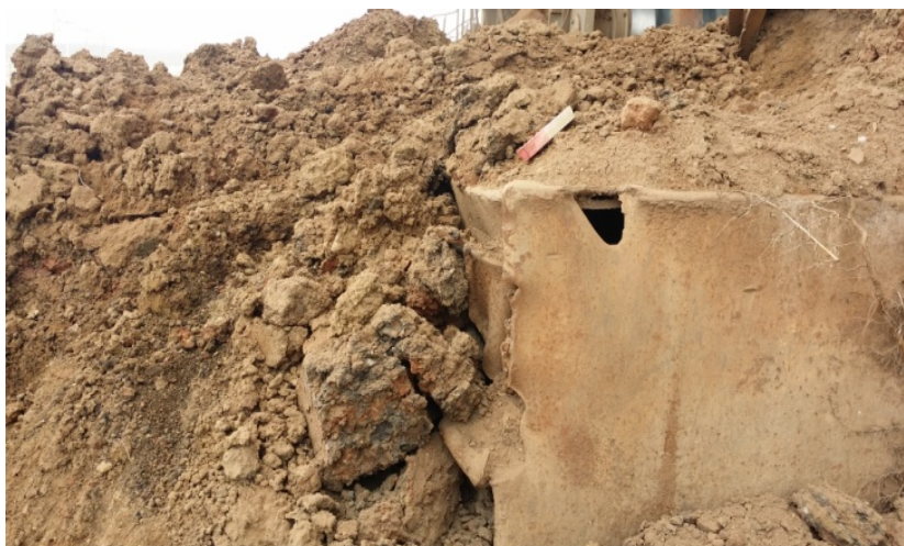
Figure 5. Damaged and covered in dried mud Drivestation's Pontoon
