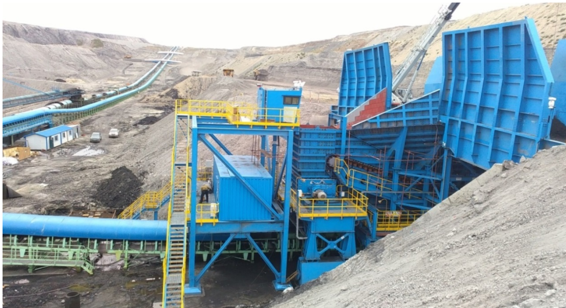
Figure 43. Semi-mobile crushing plant at YiminHe coal mine
