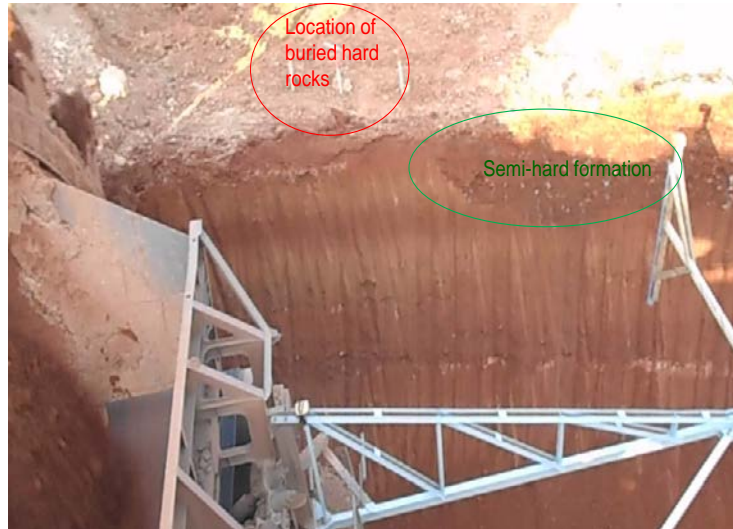
Figure 13. Photograph of the mine face during the excavation of the cut slice. The distance of buried boulders (marked with the red circle) to bench crest was approximately 0.5m. Also the occurred semi hard formation (marked with the green oval) is shown.
