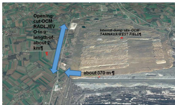
Figure 8. Correction of the opening cut position.
