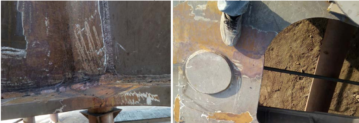
Figure 6. Geometry faults observed during inspections
