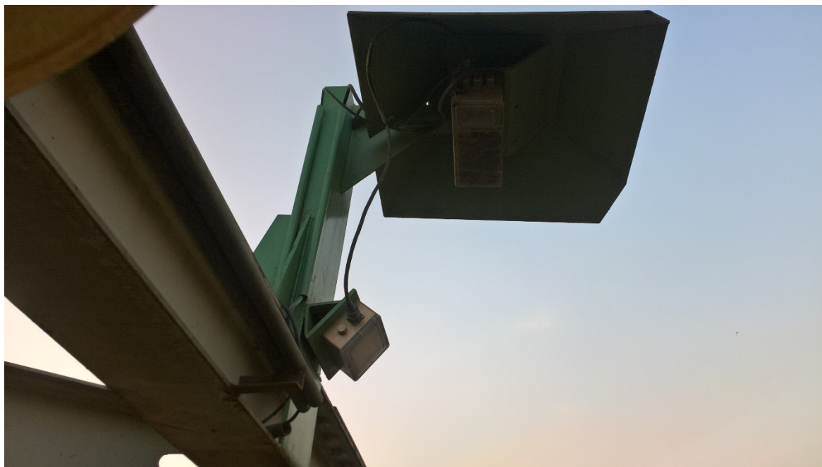
Figure 6. Installation of with iDRR and iDVR
