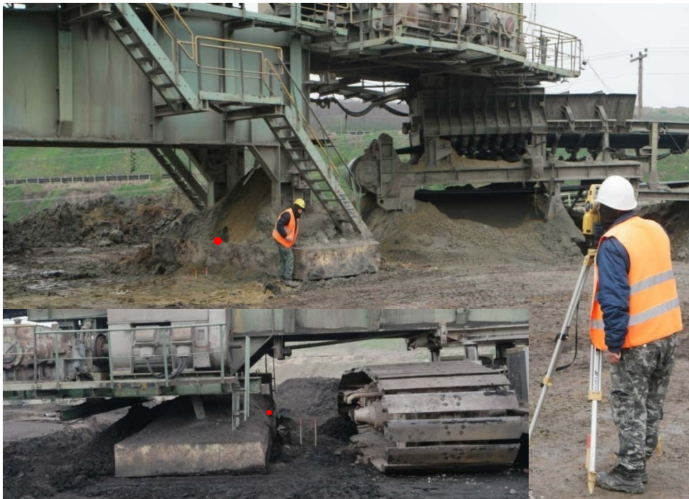
Figures 10, 11. Final staking out of the drivetrain's pontoons new positioning with laser beam guidance
