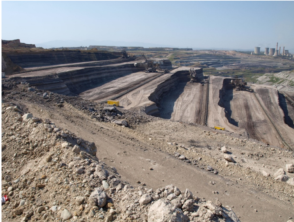
Figure 112. Typical exploitation of mine slopes using large bucket-wheel excavators and conveyor belts. Continuous advance of the slope requires a sequence of benches (60-120 m wide) and drops (15-25 m high), having an overall inclination (v:h) between 1:4 and 1:7. The figure shows five, 25 m high benches in the upper steriles of the Mavropigi mine in the Ptolemais Field.
