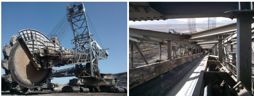
Figure 1. The PPC South Field lignite BWE (left) and detail shot of the conveyor belt (right)
