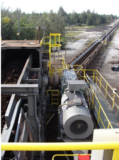
Figure 1. Typical conveyor drive with gearbox.
