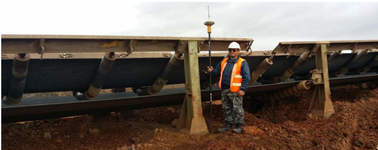
Figure 2. Each conveyor belt in WMLC’s Mine II was surveyed with dual frequency GNSS receivers in 120 epochs for optimum Real Time Kinematic accuracy, in 50m intervals of the belts
