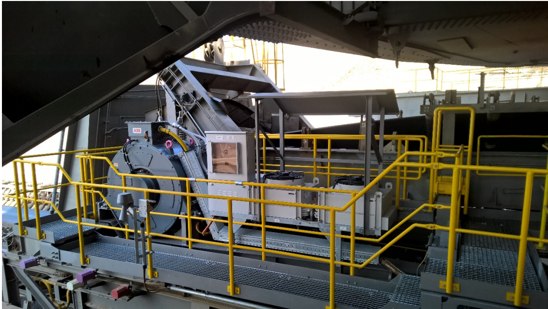
Figure 7. The GCD package at the pilot project
