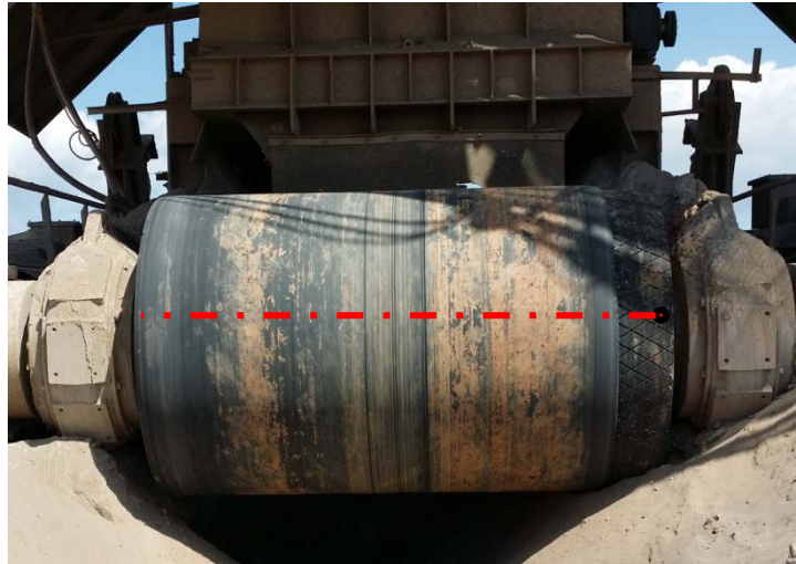
Figure 6. Tailstation drum not fully clear due to conveyor belt misalignment
