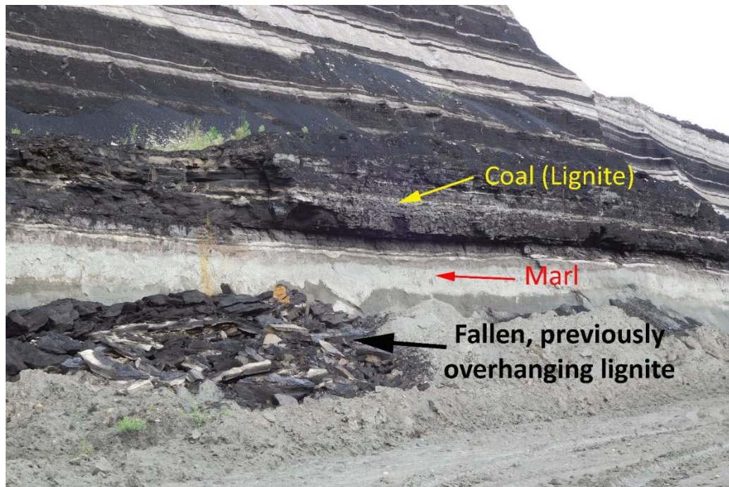
Figure 113. Critical lignite-to-marl interface close to the base of the slope. The coal expands horizontally more than the underlying marl (due to tension cracking) and overhangs the underlying marl. When the overhang exceeds the bending capacity of the lignite cantilever, the coal breaks and falls at the toe of the slope (left part of Figure).
